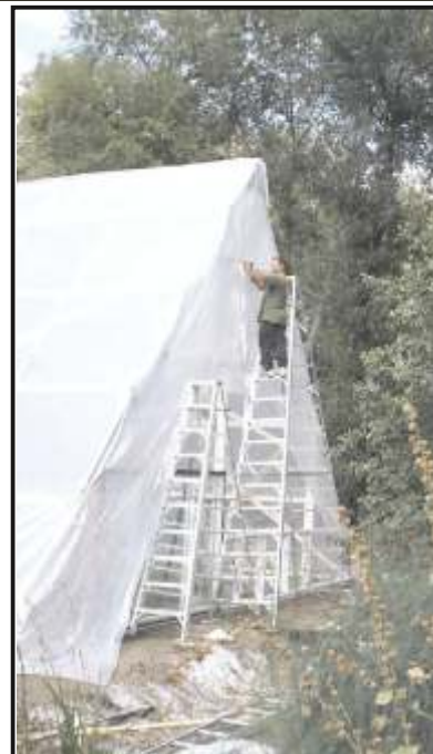
Willie attaches poly to our A-frame in September 2006. Glass windows on the lower third of the east end let us see who is entering the yard.
