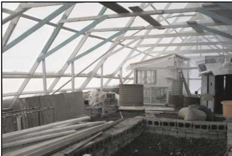
Interior of A-frame, still under construction, showing small interior starter greenhouse, which warmed up to 68 degrees F inside, by solar heat alone, despite the wind-chill factor outside, and the ice on the inside walls of the big A-frame. This will allow us to start seedlings earlier in the spring and heat only at night. We may find that we can simply cover the seedlings at night in spring and not have artificial heat out there at all. See article.
